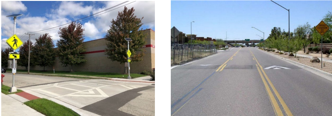
Figure 25. Raised crosswalks with speed tables and speed cushions are examples of vertical shifts that reduce operating speeds
