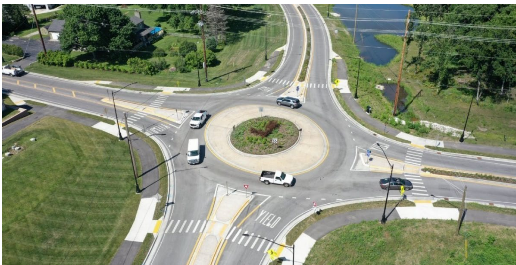
Figure 24. Roundabouts and traffic circles are examples of horizontal curves that reduce operating speeds
