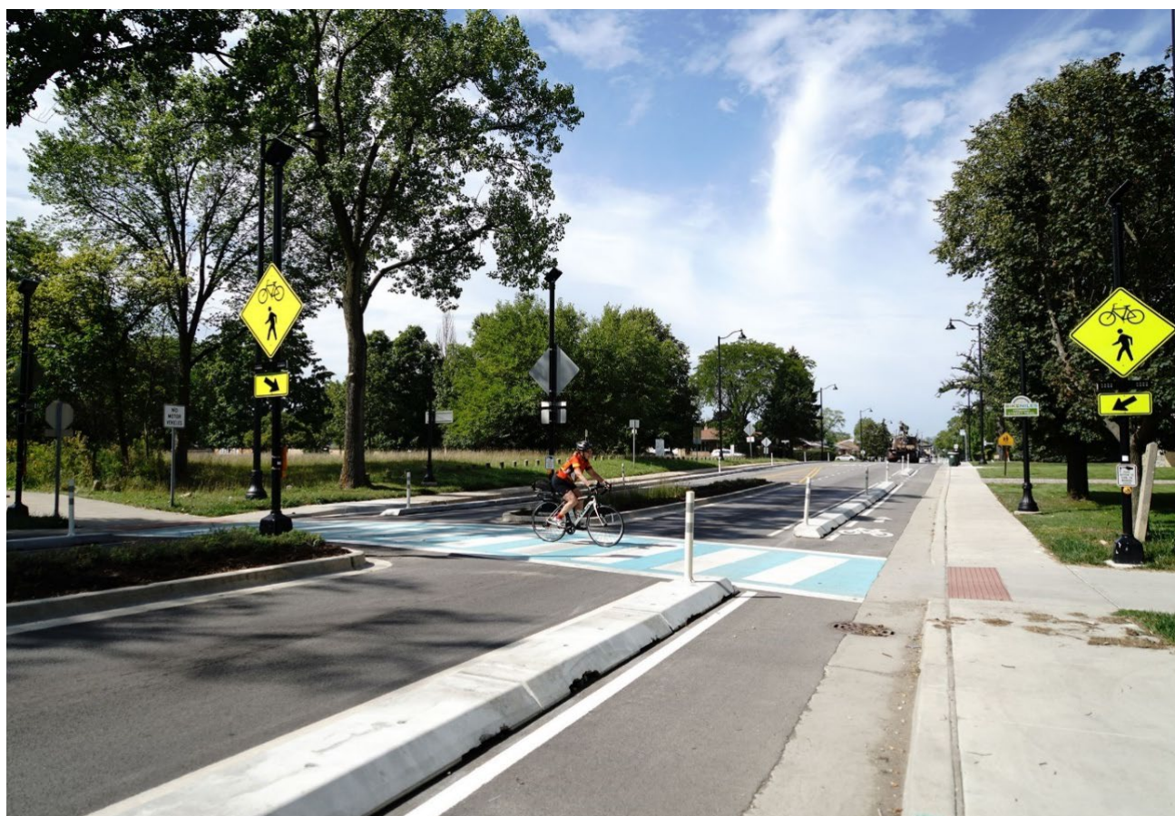
Figure 23. A road diet with a planted median in Niles, Illinois, improved safety by reducing the width of the roadway and slowing vehicle speeds with visual friction
